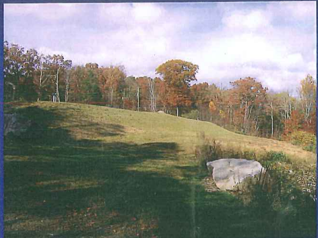
Large Scale Subsurface Wastewater Absorption System Post Construction - Subsurface Wastewater Absorption System Area
