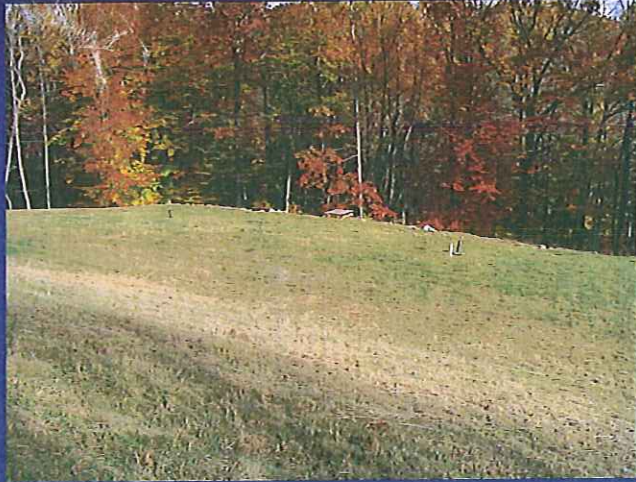
Large Scale Subsurface Wastewater Absorption System Post Construction - Subsurface Wastewater Absorption System Area
