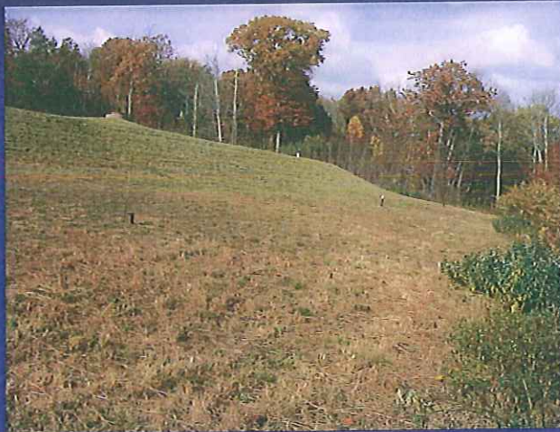
Large Scale Subsurface Wastewater Absorption System Post Construction - Subsurface Wastewater Absorption System Area
