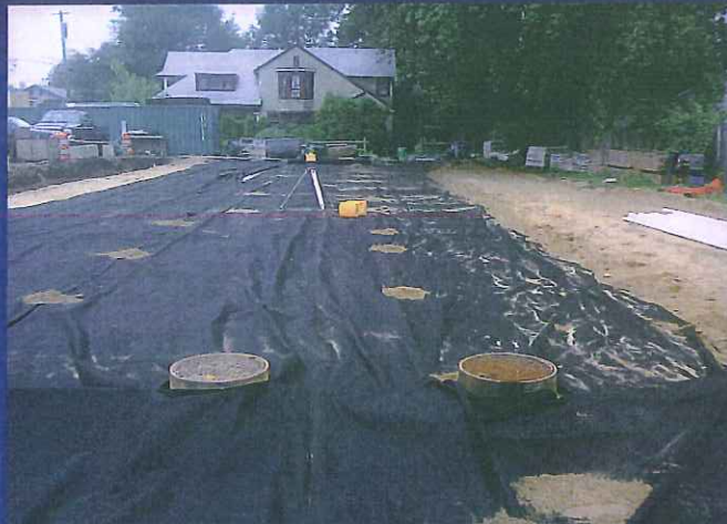
Large Scale Subsurface Wastewater Absorption System Construction - Covering System with Fabric
