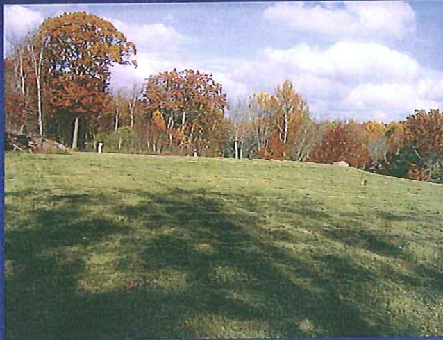
Large Scale Subsurface Wastewater Absorption System Post Construction - Subsurface Wastewater Absorption System Area
